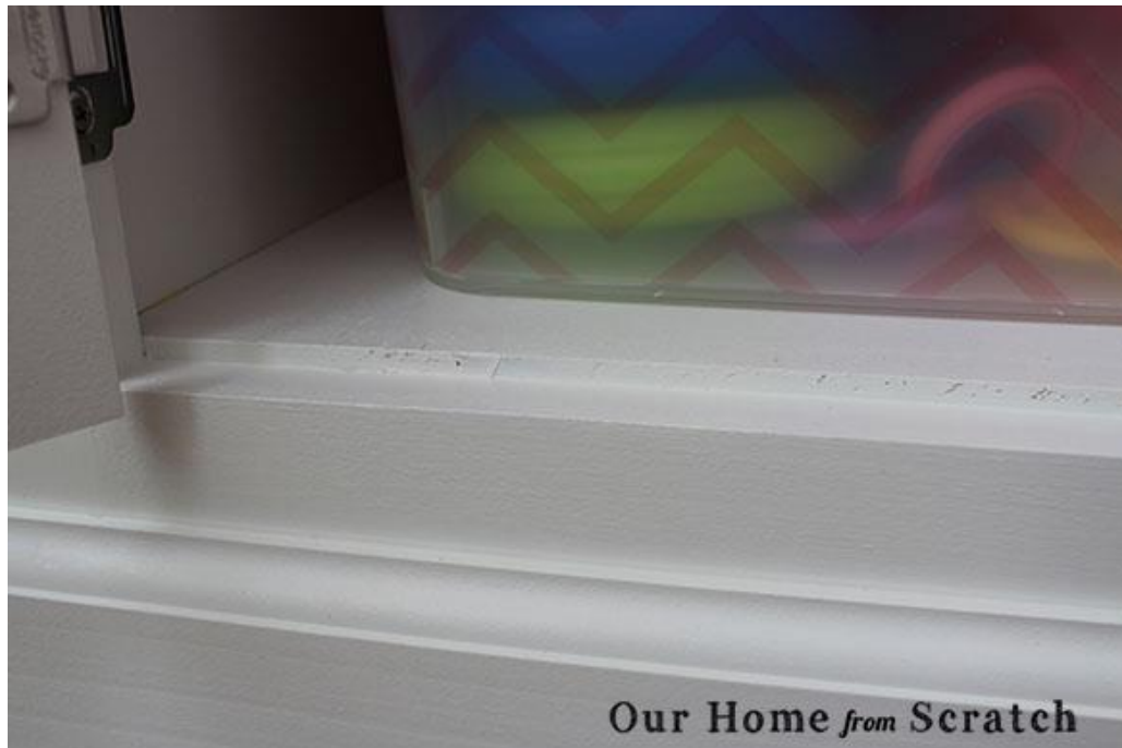
Figure 13: Bottom Board Extends Above the Top of the Face Frame
